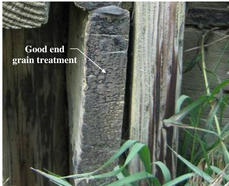
Figure 4-14. Good backwall with treated end grain
