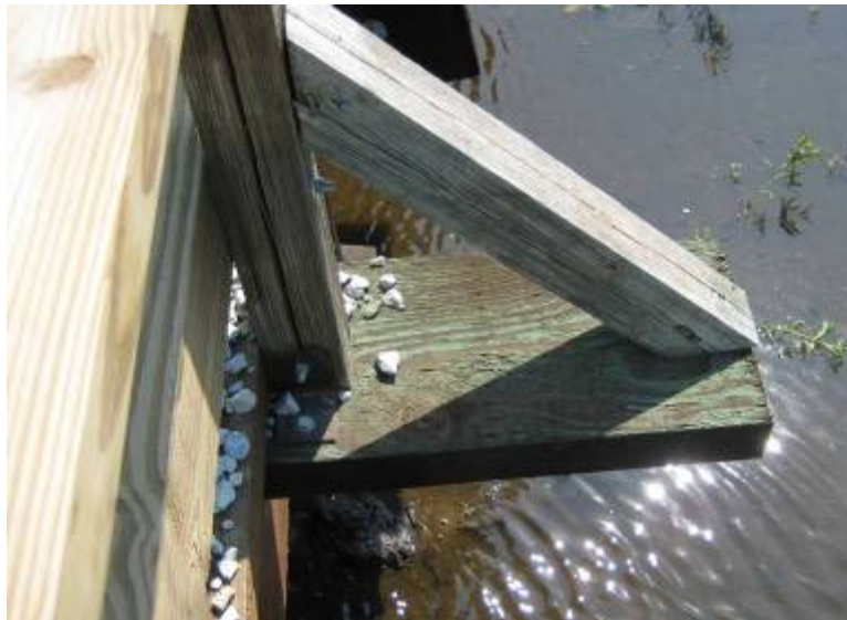
Figure 4-52. Top side of cantilevered copper naphthenate-treated decking
