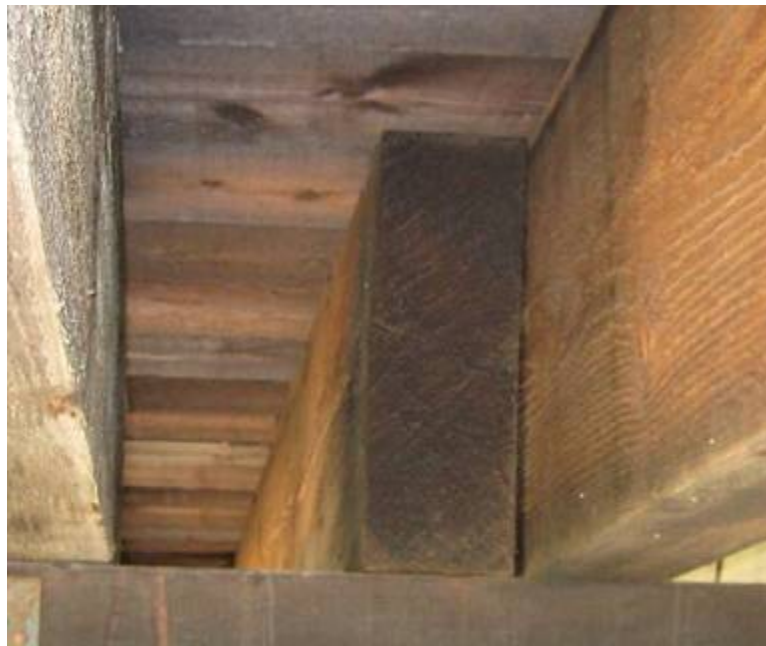
Figure 4-36. Stringer end grain with good treatment and no visible decay
