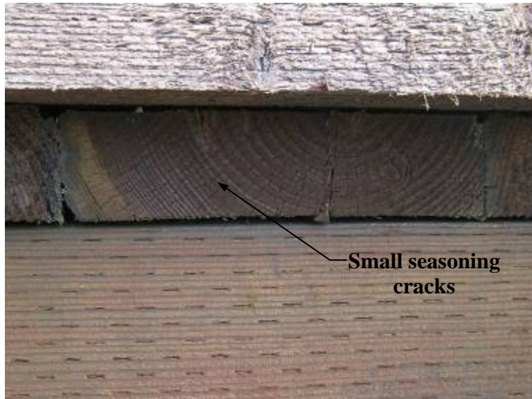
Figure 4-53. Good end grain of copper naphthenate-treated bridge deck
