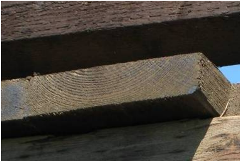
Figure 4-39. Treated bridge deck with excellent preservative treatment and member condition
