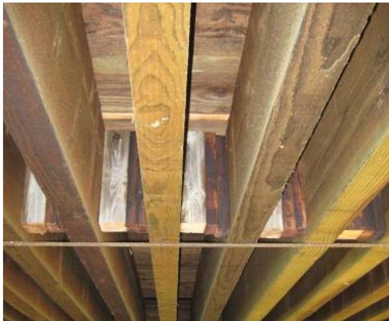
Figure 4-49. Good copper naphthenate-treated stringers
