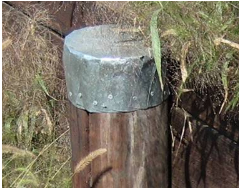
Figure 4-9. Good metal pile cover to prevent pile top decay
